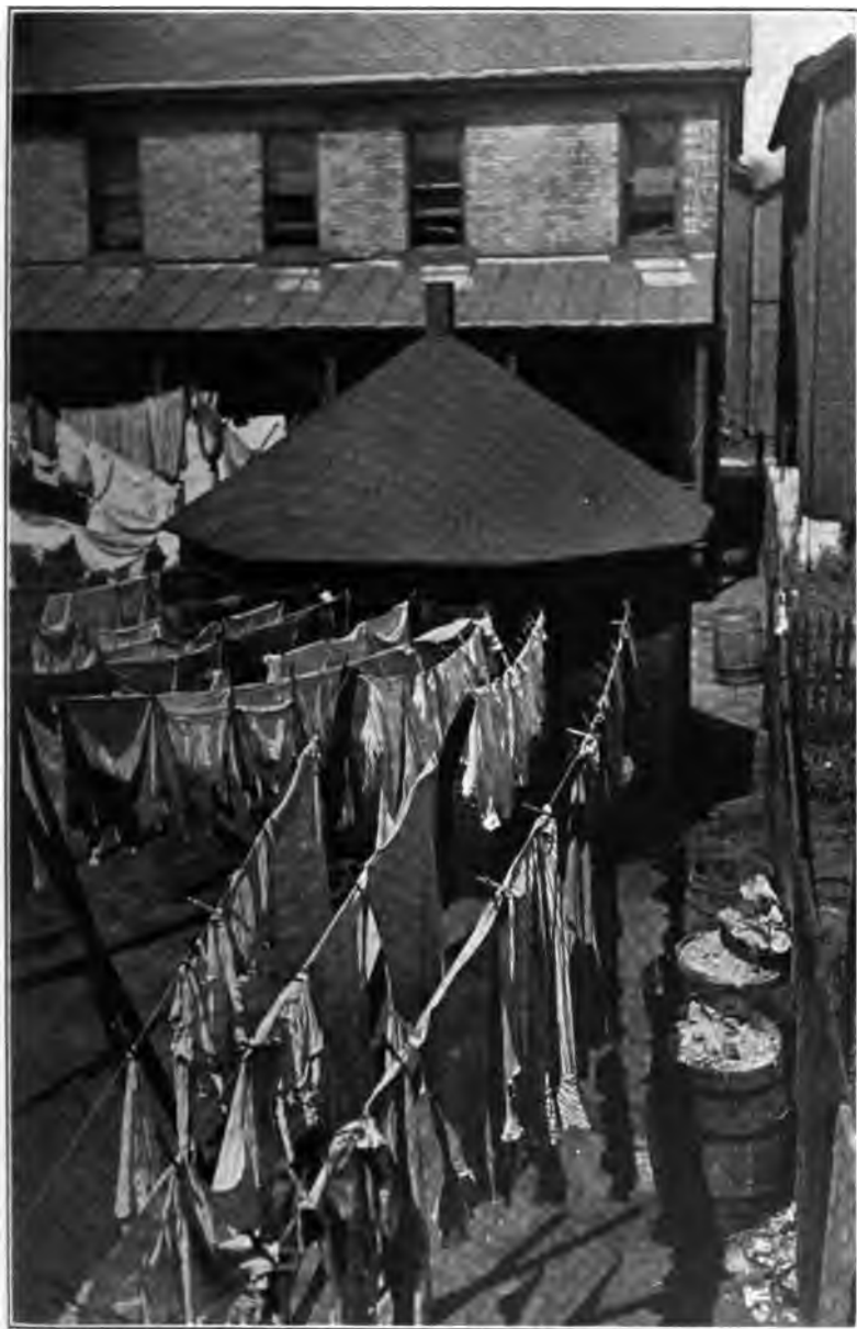
WASH DAY IN AN INNER COURT, BRADDOCK Thirteen families used this court. In the octagonal building eight closets emptied into a sewer which was flushed only occasionally
